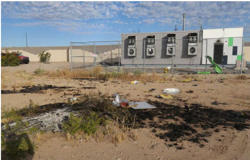
Figure 4.19: Photograph of burned bush, E193 Capt's helmet, and SCBA tank removed during the deflagration [6].
