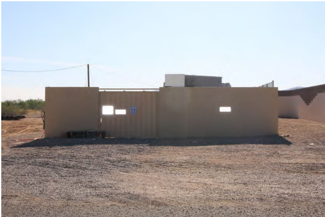
Figure 4.2: Photograph of the solid wall and gate to the northeast of the ESS [13].
